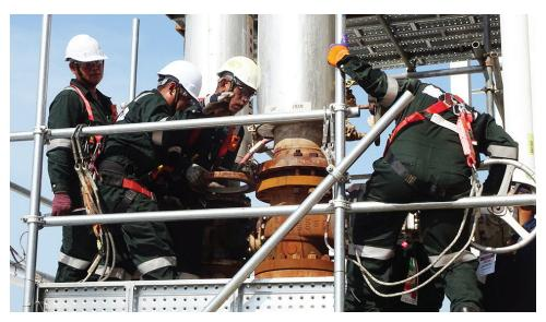
Hot bolting is the practice of sequential removing and replacing of bolts on a bolted joint (e.g. flange, heat exchanger, manway, etc.) while the joint assembly is under reduced operating pressure. This practice is potentially hazardous, and the utmost caution, therefore, needs to be exercised and carried out while under permit and controlled conditions. In many documented accidents where hot bolting has failed, there have been fatal casualties, fire, explosion, and loss of equipment and plant.
